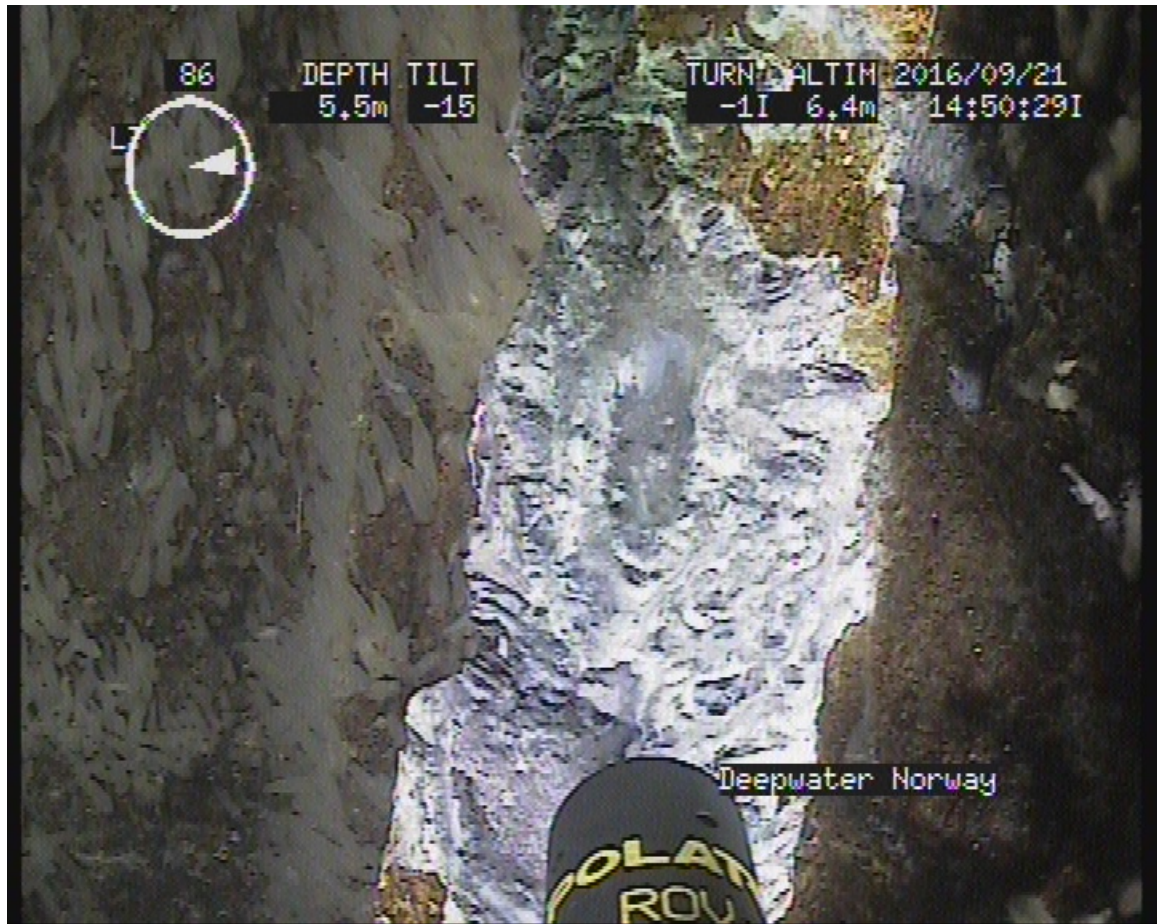
Figure 6-2 Picture of cleaned anode showing large pits and hard marine growth outside the jetted area
