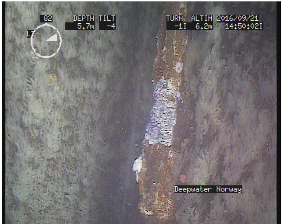
Figure 6-1 Picture showing sheet piles with marine growth and anode with cleaned section
